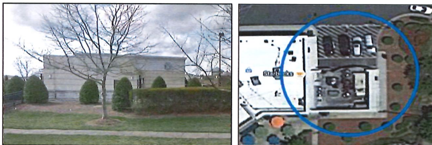
Figure Set 17: Acceptable Service / Loading Area Screening Along Roadways (Blakeney, NC)
