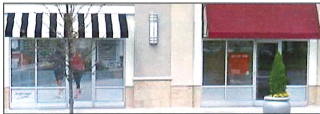
Figure 08-09: A Model of Acceptable Window Films Pursuant to Standards and Design Review & Approval.
