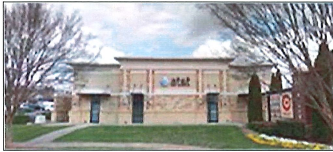
Figure 03: Rear-side of building public-right-of-way Featuring faux façade with transparent windows & doors
